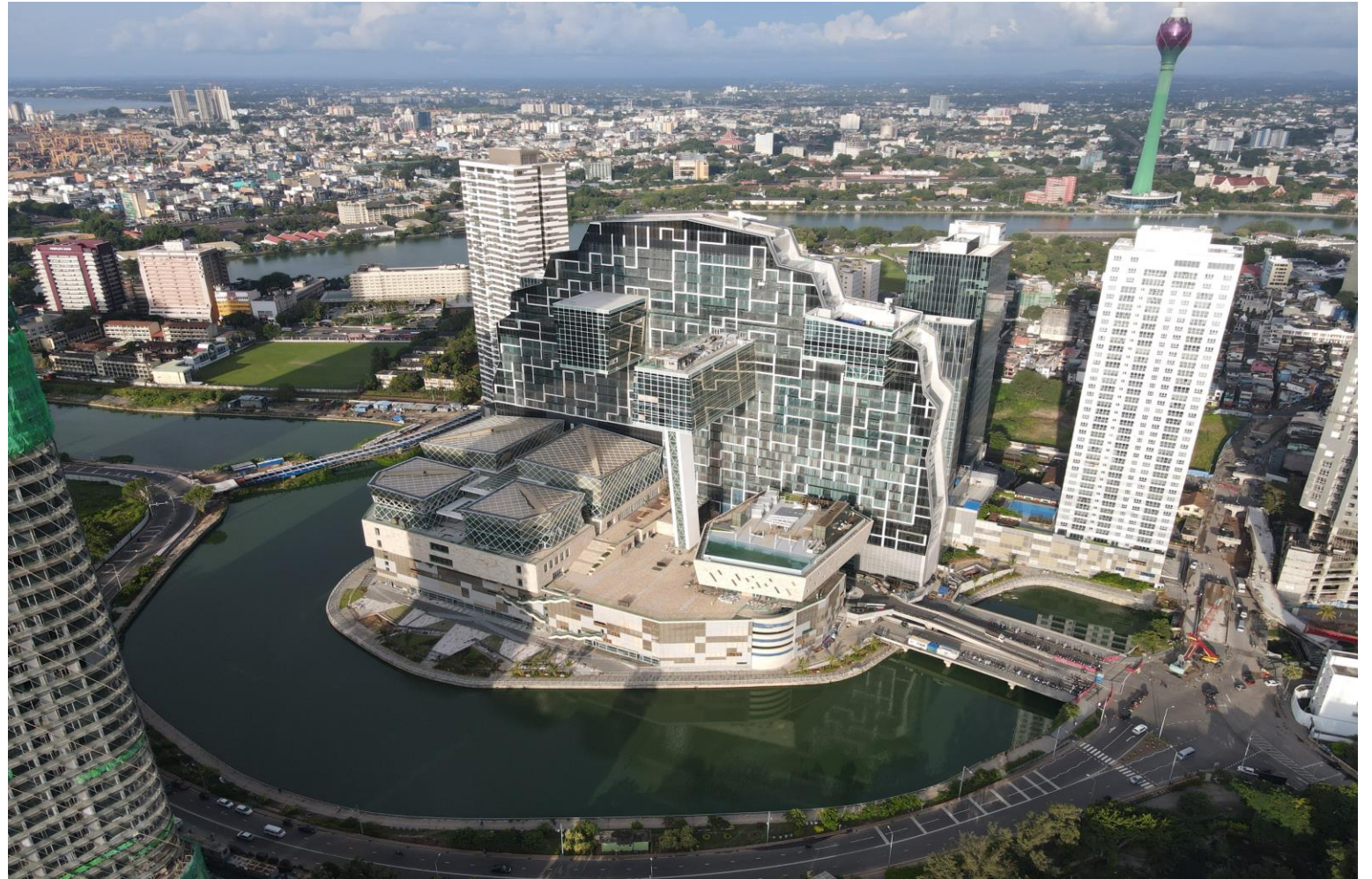
“Cinnamon Life” under construction
