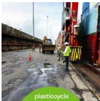
PMAC road resurfacing project at SAGT
