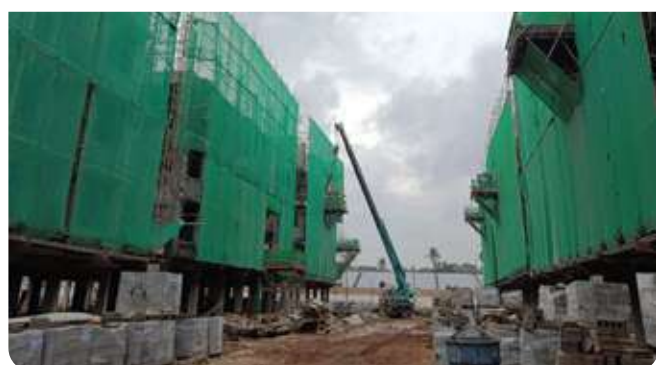
VIMAN - structural completion of both phase 1 and phase 2.
