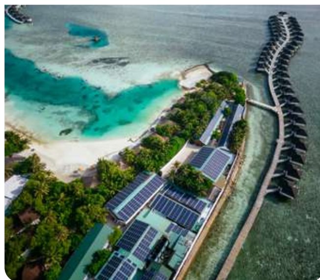
Solar panel installation at Cinnamon Dhonveli Maldives.
