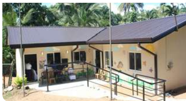
Newly constructed Nithulemada Pre-School.
